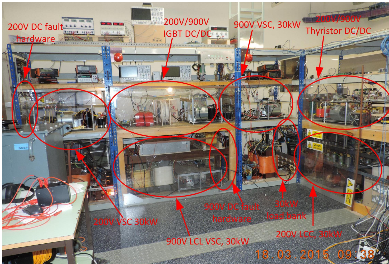
Figure 33. Aberdeen DC test grid. 4 AC/DC converters and 2 DC/DC converters
