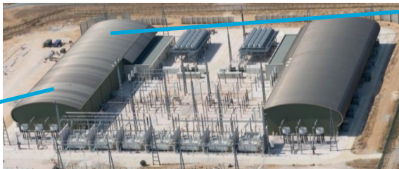
Stations de conversion
